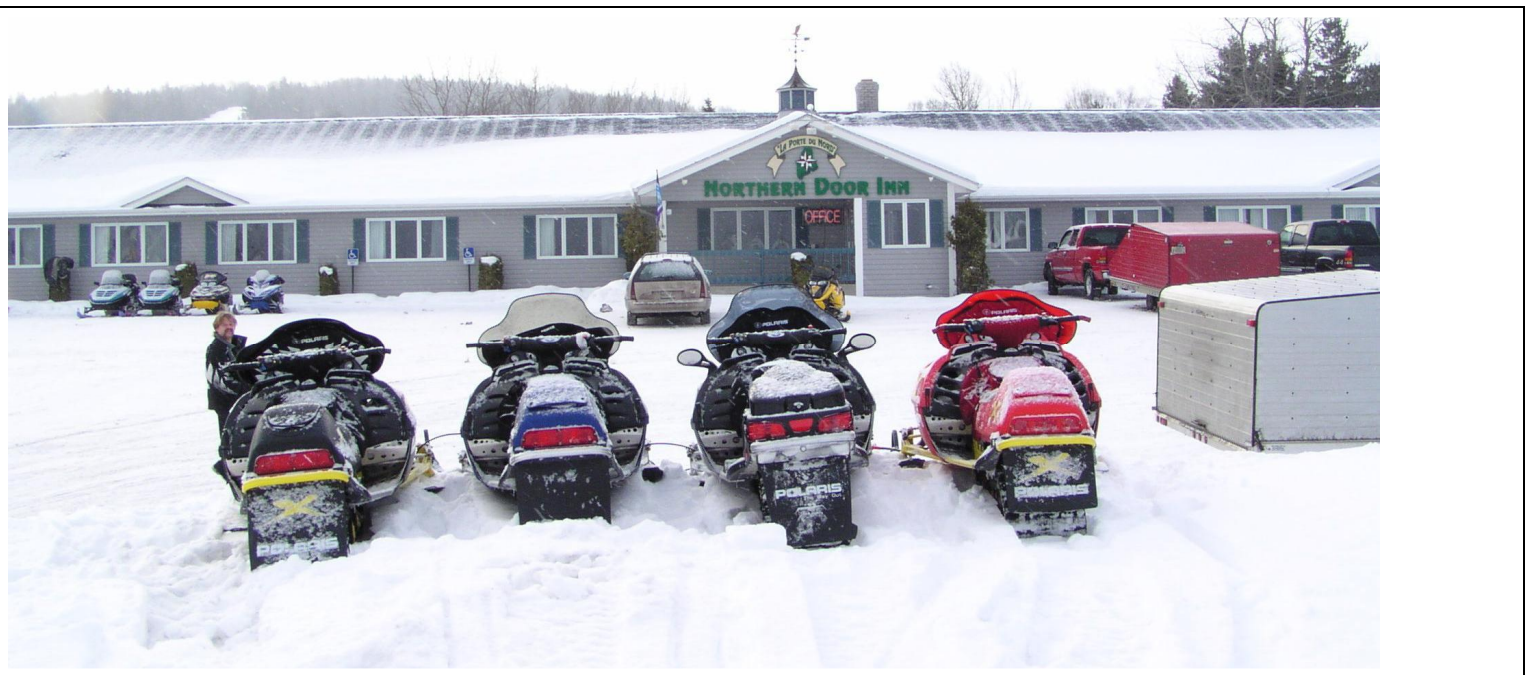
Northern Door Inn, Fort Kent
